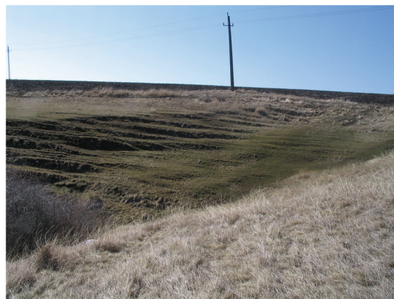
Fig. 12. Landslides in Bogács
